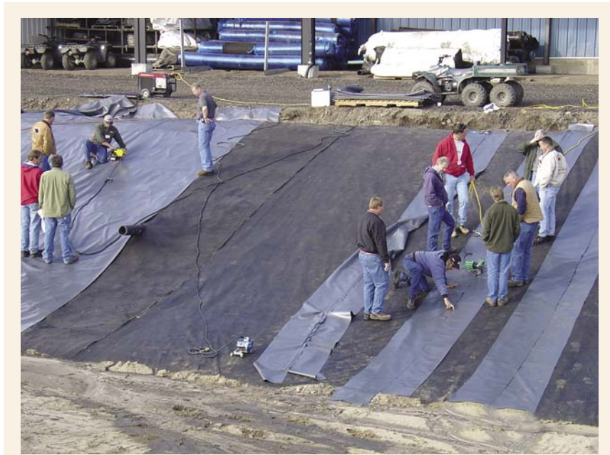
Photo 1. Wedge welding and air-channel testing area at the PGI workshop.
