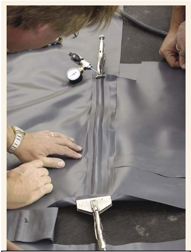
Photo 3. Air-channel testing of T seam in 30 mil sheet.
